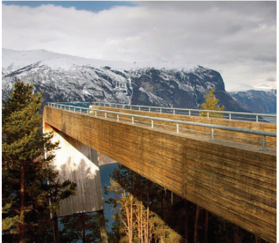
Stegastein Viewpoint overlooks the Aurland Fjord from 650 metres. It was designed by Canadian architect Todd Saunders with Norwegian architect Tommie Wilhelmsen as part of the National Tourist Routes initiative.
