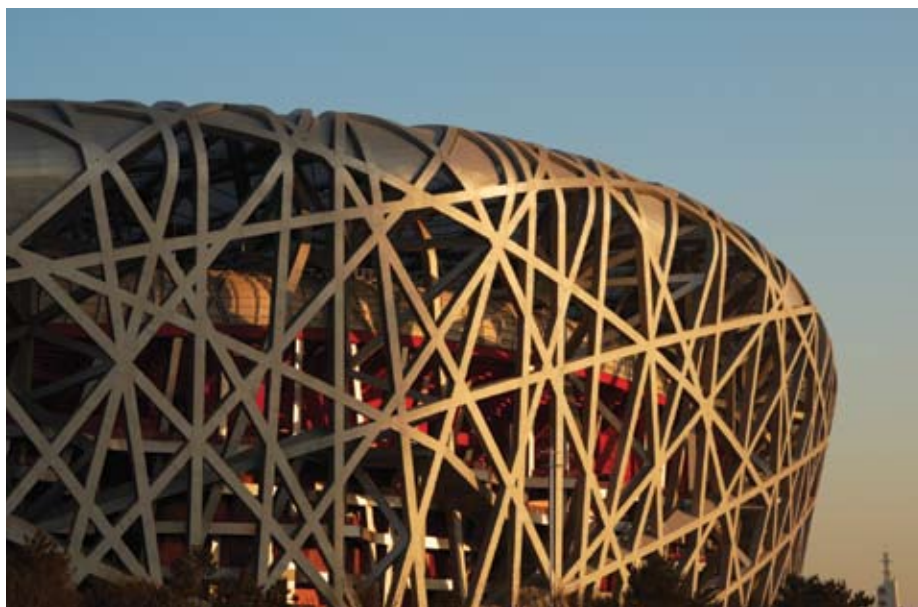
The China National Stadium, also known as the "Bird's Nest," will serve as the main stadium for Olympics.
